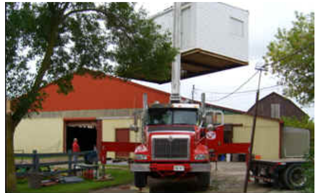
Over works better than under
